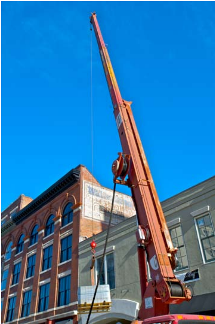
A construction crane lifts a pallet of tiles to the roof of a building located on the Commerce Street side of The Alley in downtown Montgomery.
